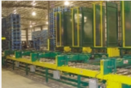
Specialized pallet sortation equipment is utilized in many of our operations. This equipment is acquired and maintained by Amware as part of our agreement with our customer.
